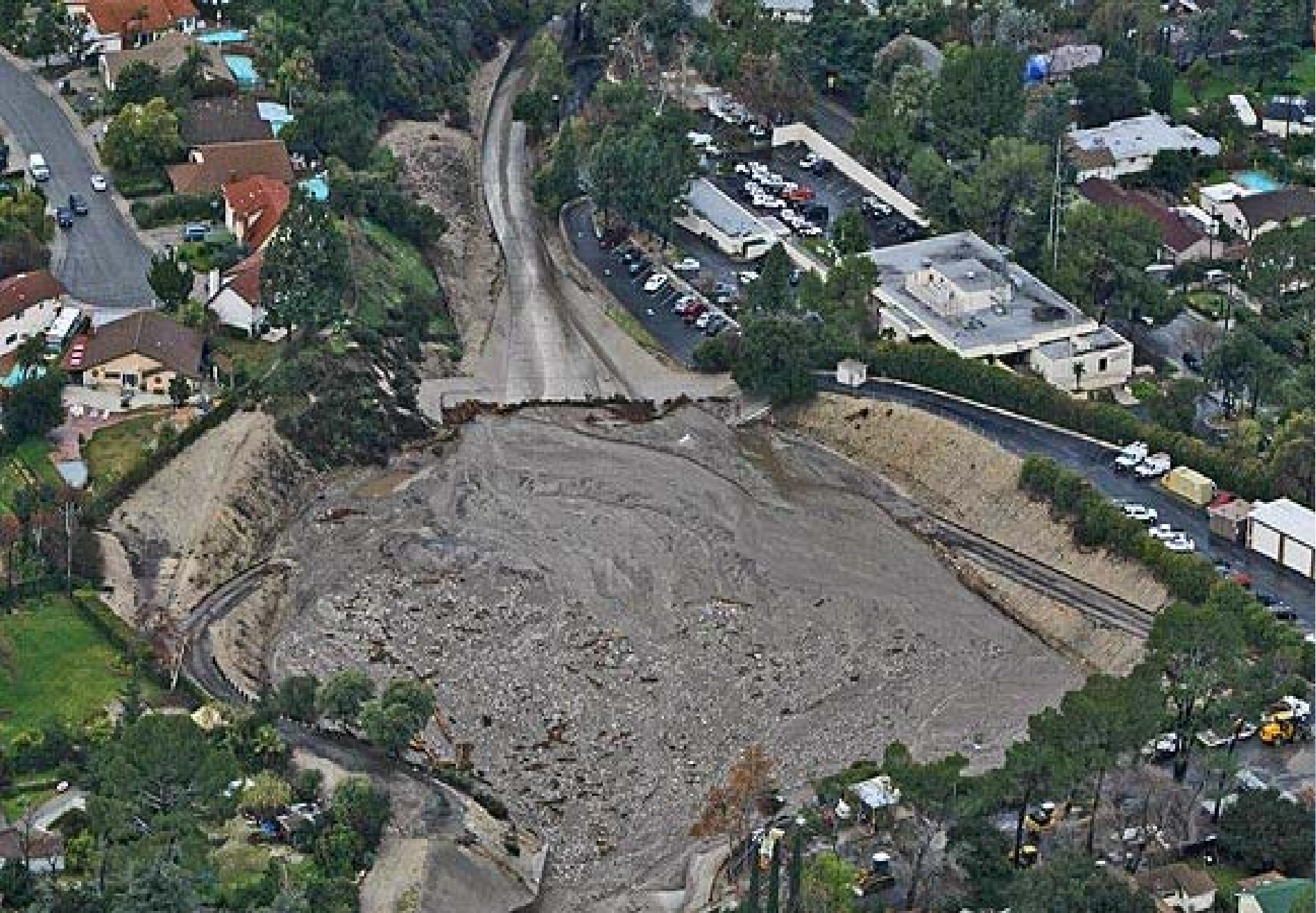
Pickens Debris Basin – 2009-10 Storm Season
